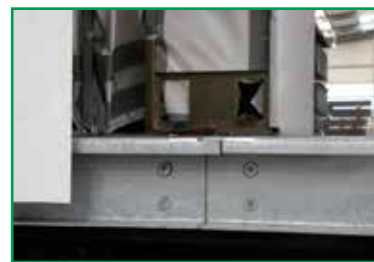
Laufschiene aus Stahl in Segmenten verschraubt Running rail made of steel, bolted in segments
